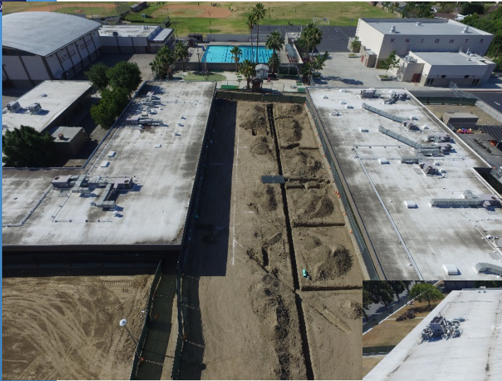
Phase A1 Hardscape demo and grading, excavation for piping.
