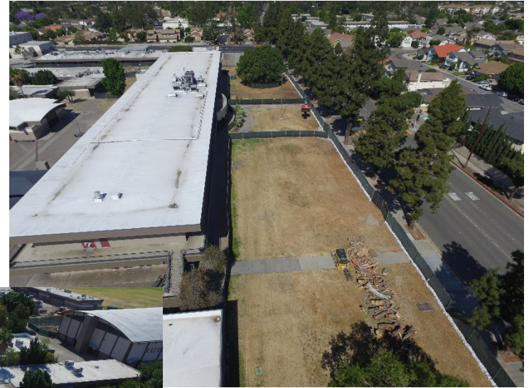
Phase A1 Landscape demo and contractor staging areas
