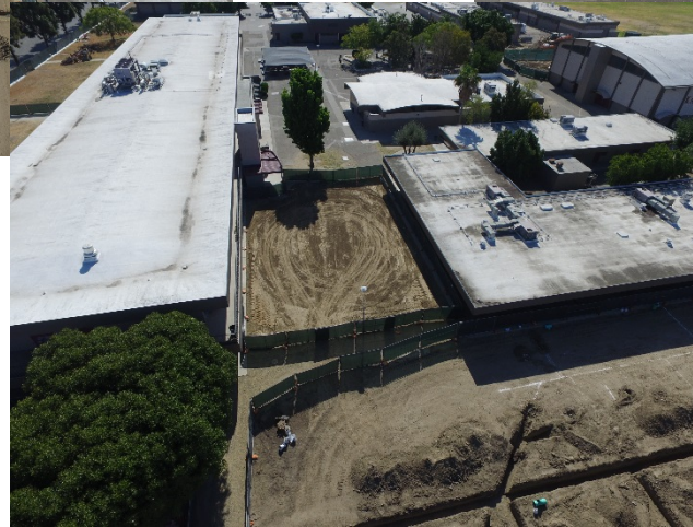
Phase A1 Hardscape demo and grading, excavation for piping.
