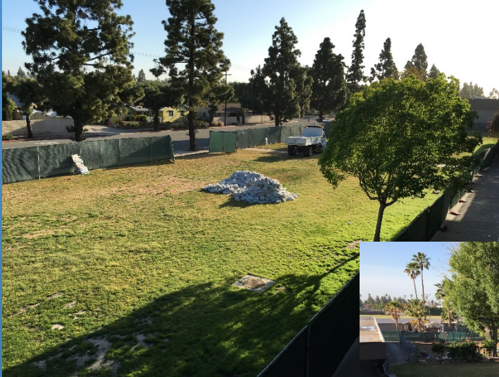
Phase A1 Start of construction in landscape area along Wagner Ave.
